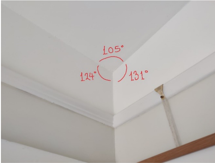
Figure 2. Not a right angle when looked at.
